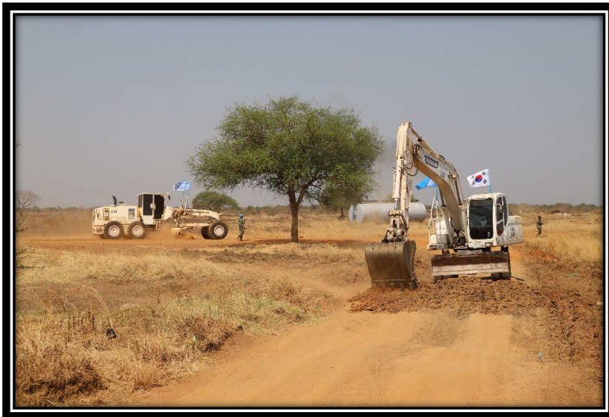
Road rehabilitation conducted by UNMISS ROK contingent in support of operations
